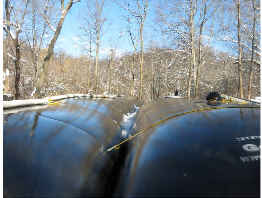
Geotubes set up at the site
