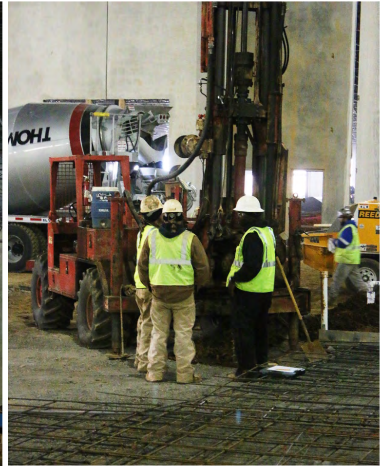
Grouting NW of Pit 12. Note the rebar for impending slab pour.
