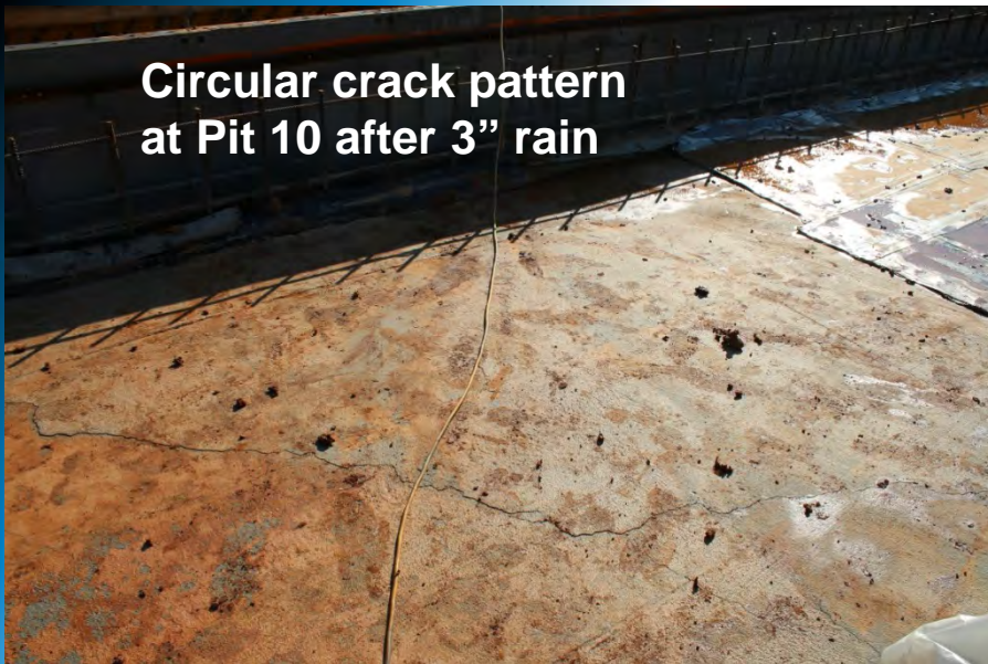
Distress at Equip. Pit 11 after 3" rain
