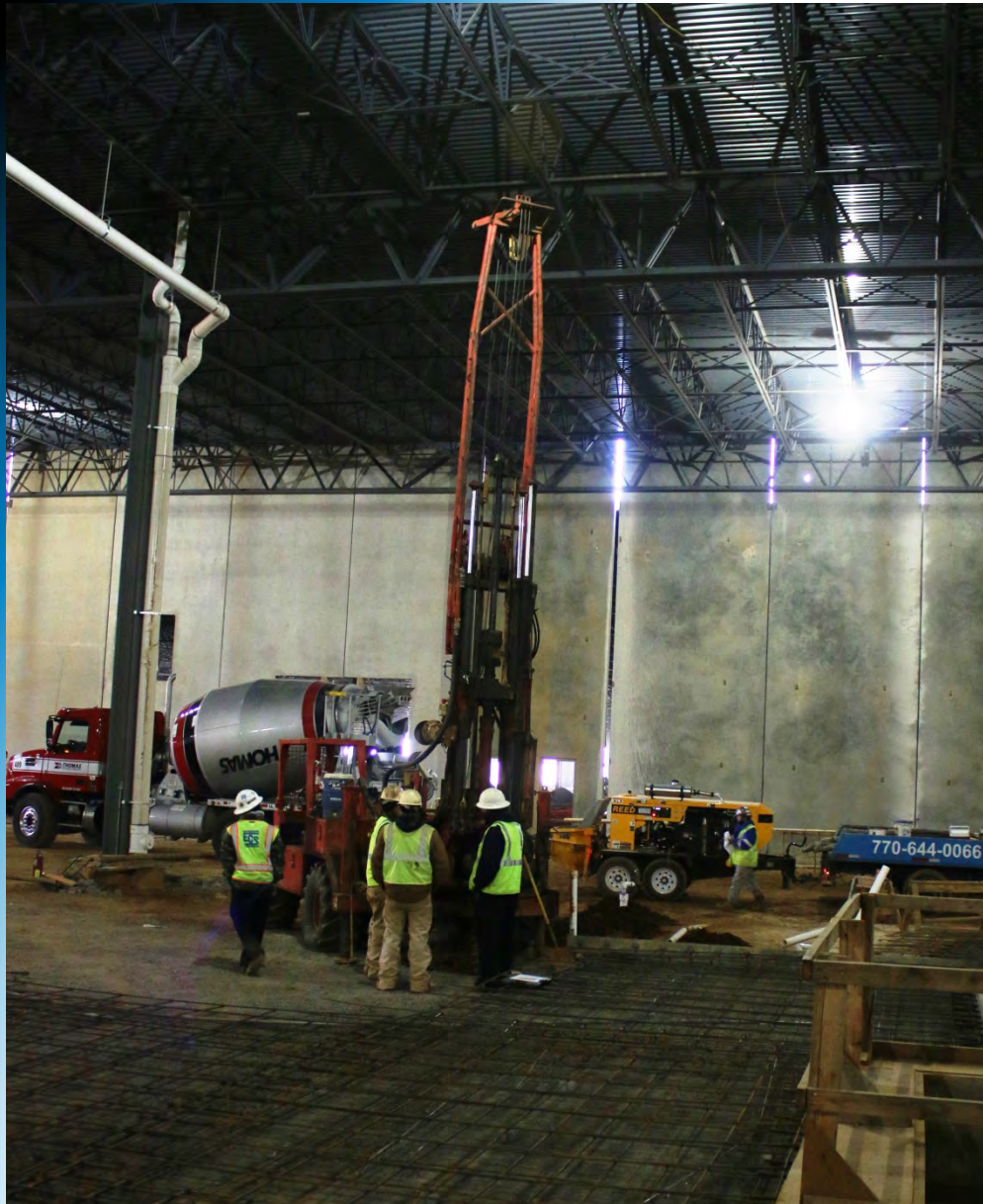
Grouting NW of Pit 12. Note the rebar for impending slab pour.
