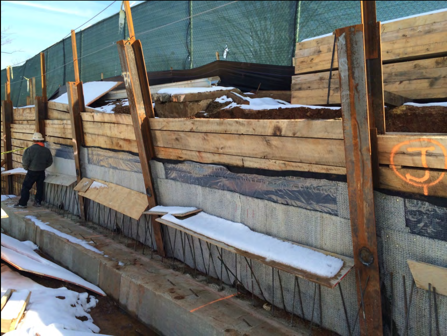
Frozen ground behind sheeting
