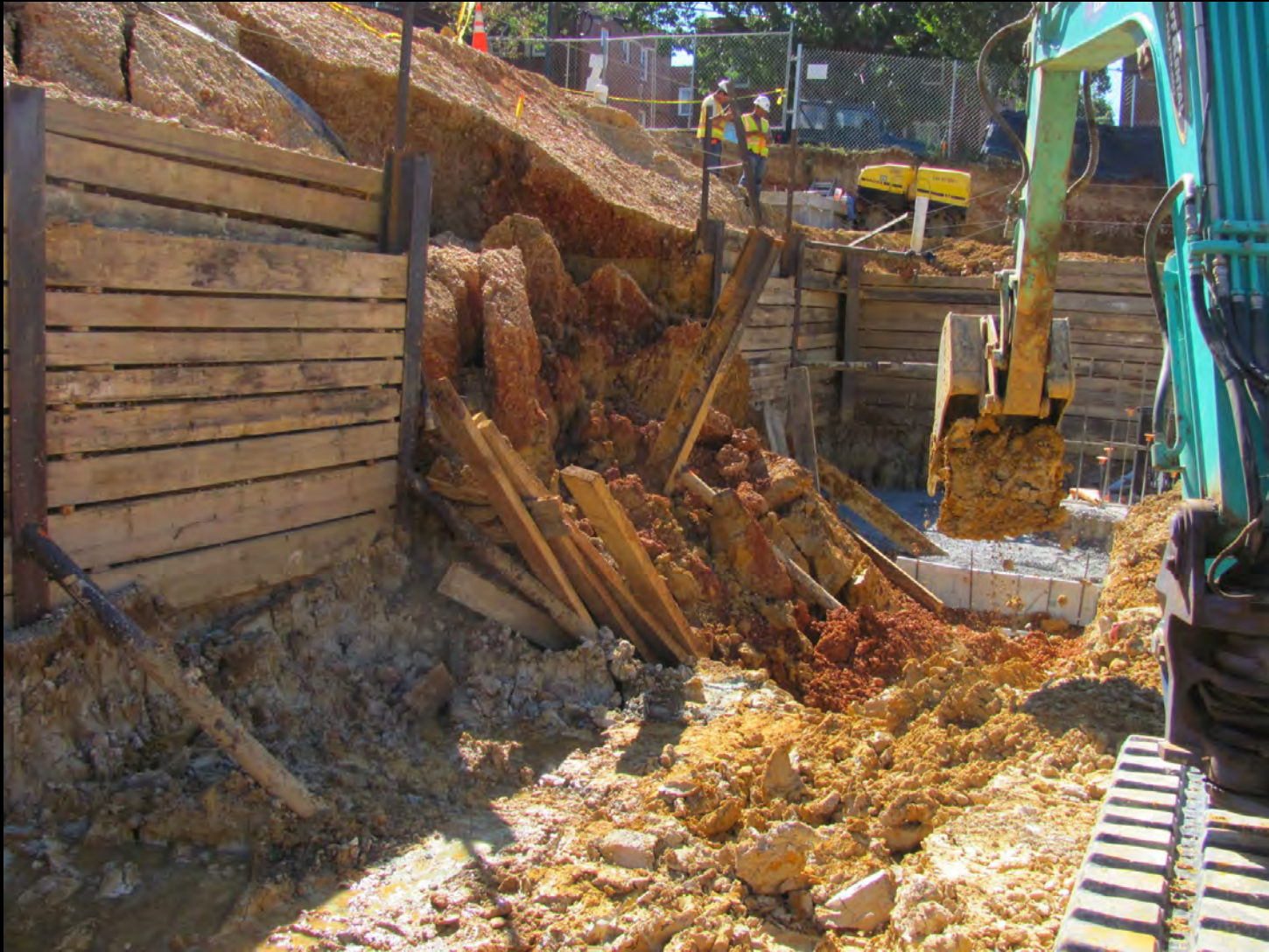
Excavation on passive side of heel block
