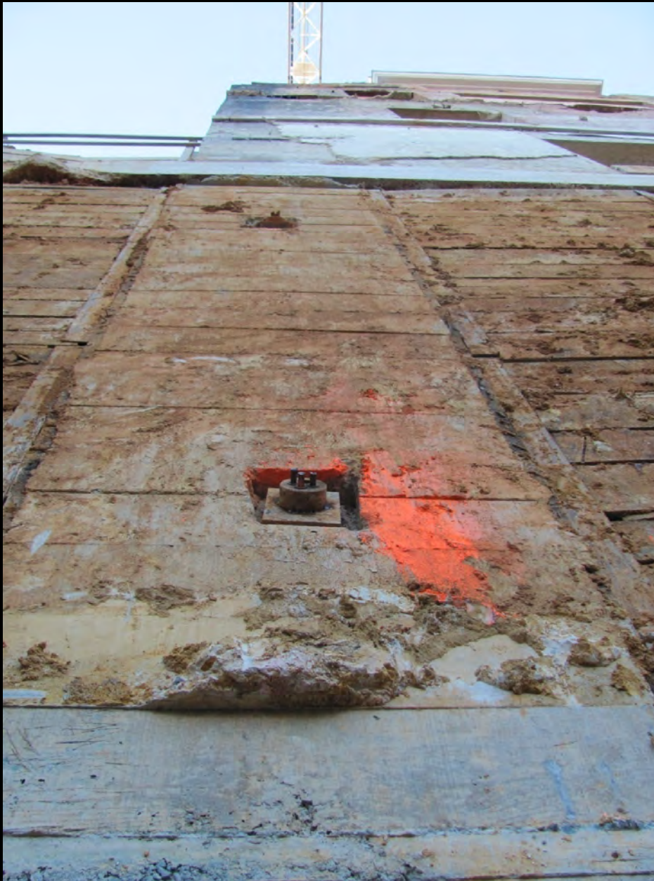
Hand dug underpinning pier supporting a church in Arlington, VA
