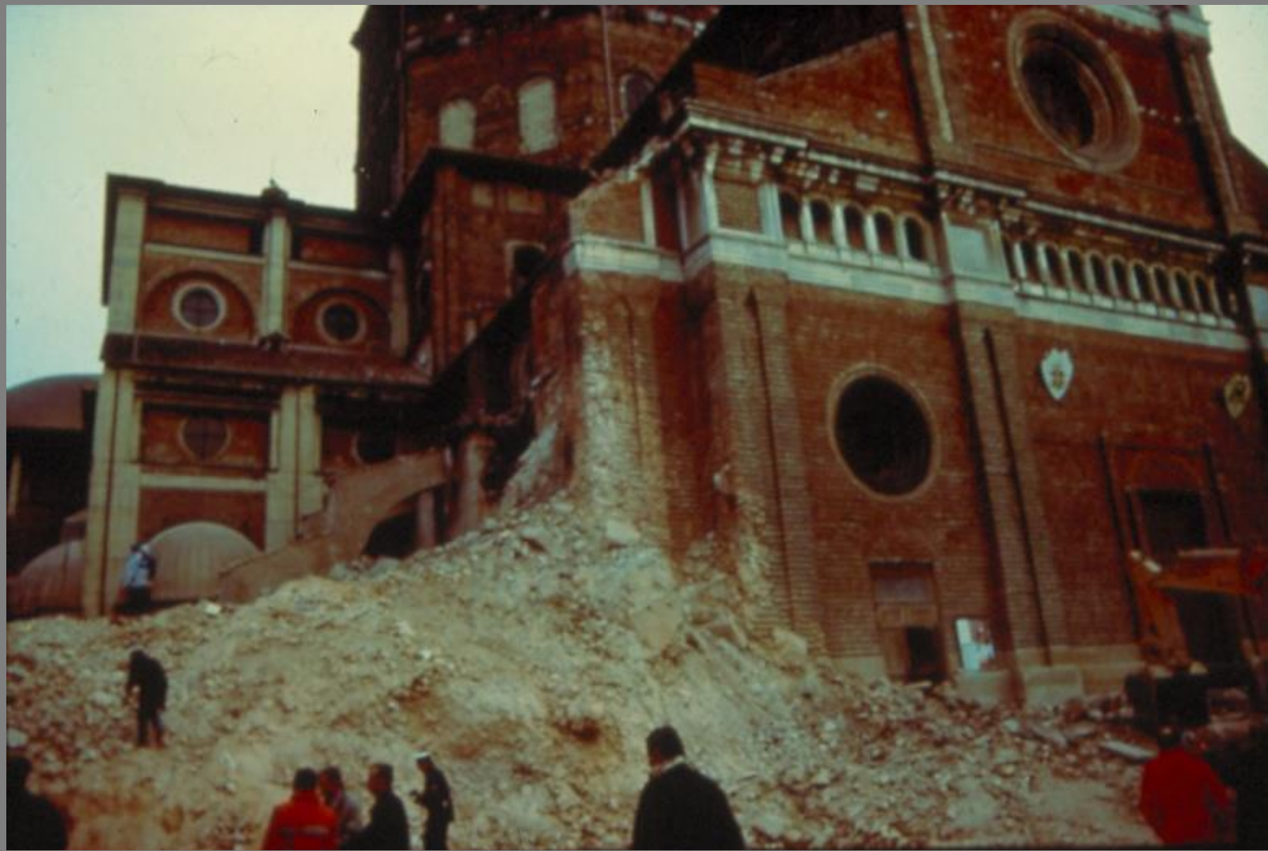
The collapse of the civic tower of Pavia, 1989
