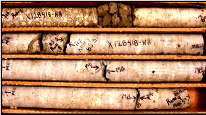
Fig. 18. Core at Caisson 69 showing 4-inch clay zone (top row) between concrete and dolomite bedrock at 84 ft.
