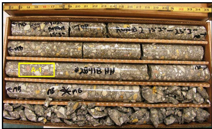
Fig. 12. Broken concrete core from approximately 22 to 24 feet at Caisson 90.
