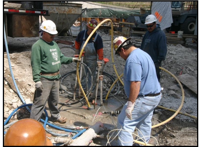
Fig. 13. Remediation pressure grouting of the shallow anomaly at Caisson 90.
