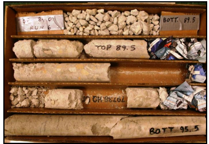
Fig. 16. Concrete core at Caisson 2 showing weak concrete, segregated concrete and gravel zones above bedrock from 84 to 93.5 ft.
