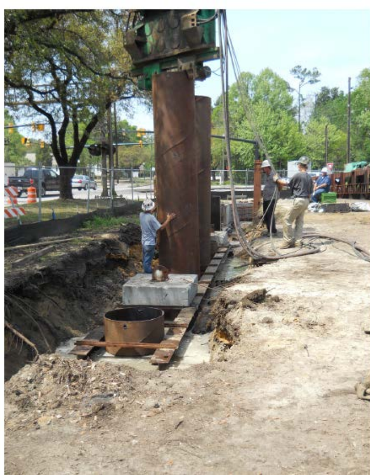
Temporary Steel Casing Installation Vibratory Hammer
