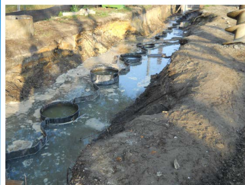
Installed System Prior to Concreting and Excavation
