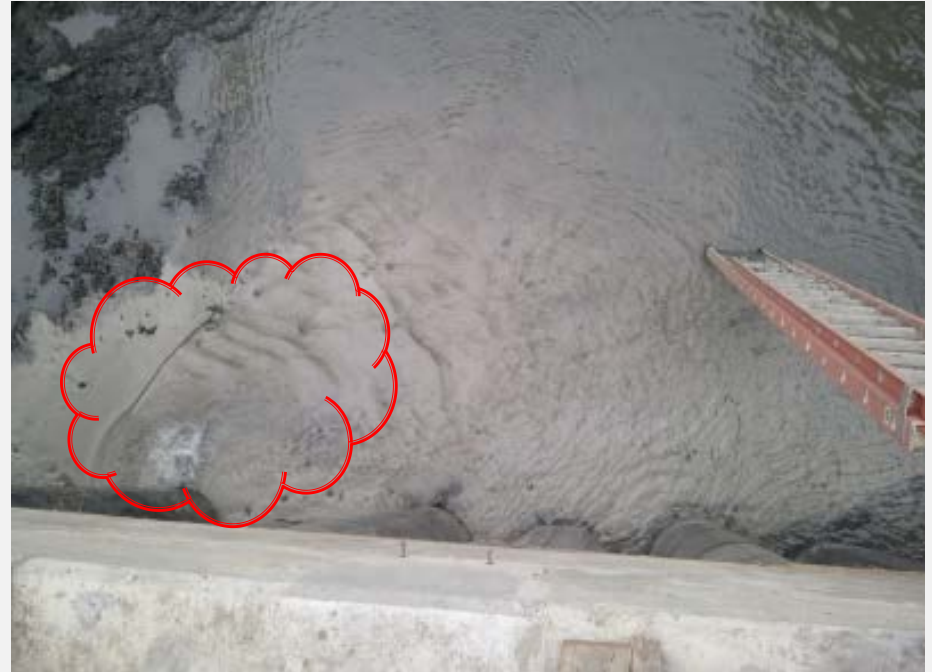
Artesian Conditions At Base of Wet Well Excavation
