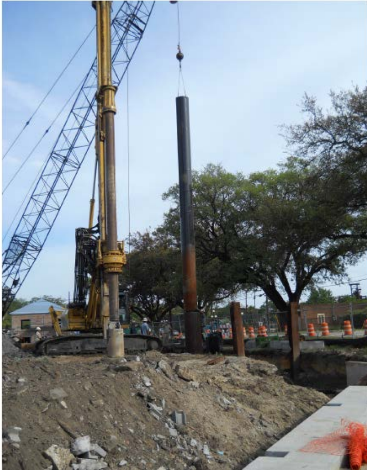
Pile Shell Installation
