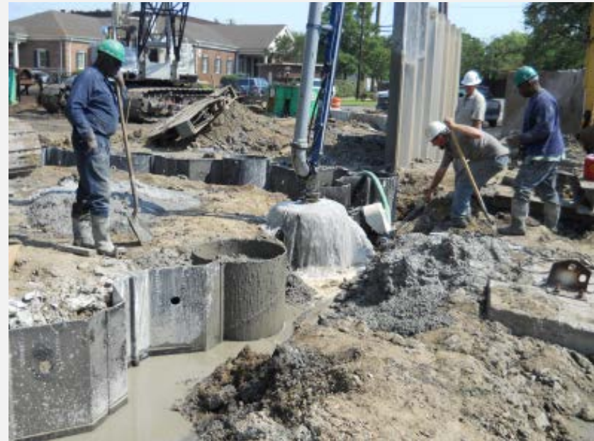
Concrete Placement Tremie Method
