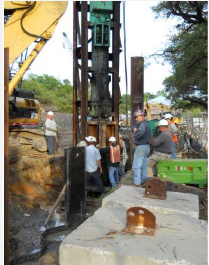
Steel Shell Driven To Design Tip Elevation
