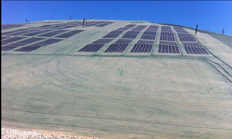
Hickory Ridge Solar Cells on Exposed Geomembrane Cover (Republic Services - Atlanta)
