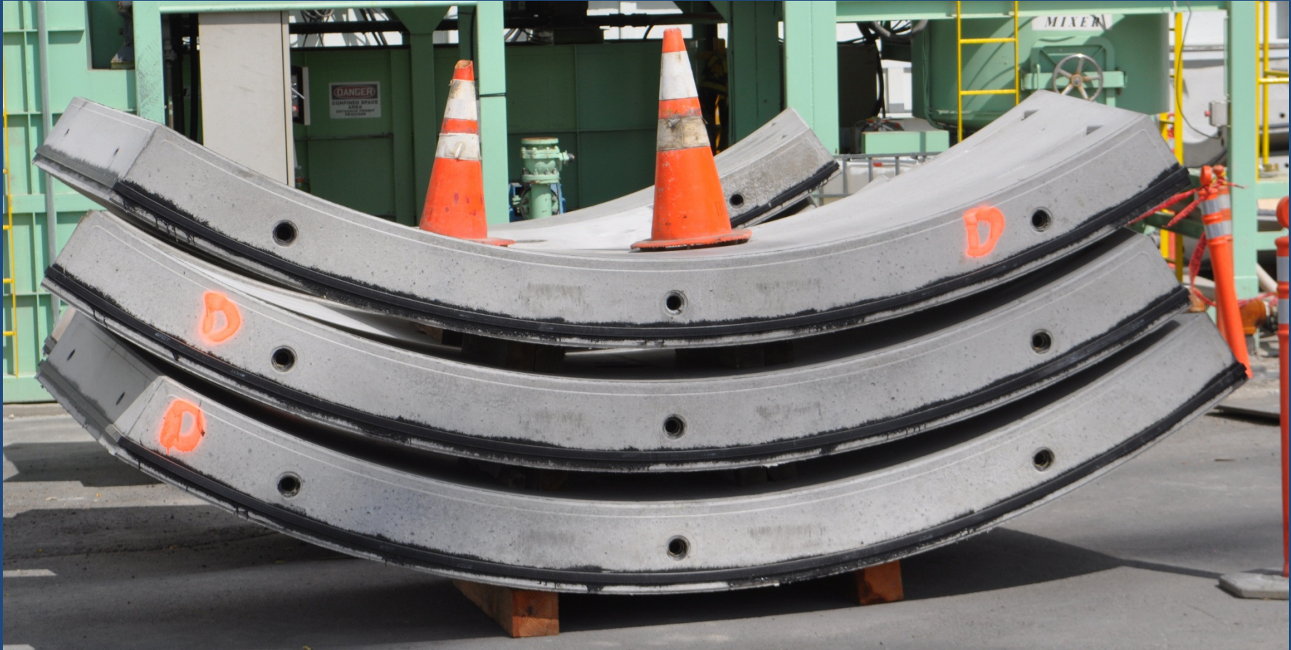
Concrete Segments, with gaskets Erected in tunnel to form a 6-piece Ring
