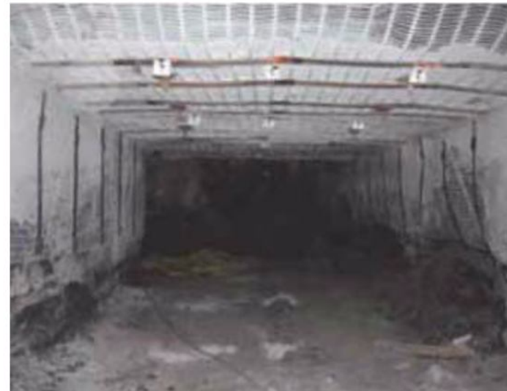
New Long Wall Mining
