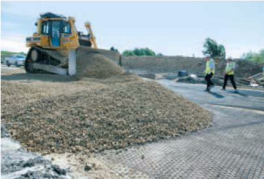
Old Subgrade Reinforcement Reinforcement Over Old Landfills
