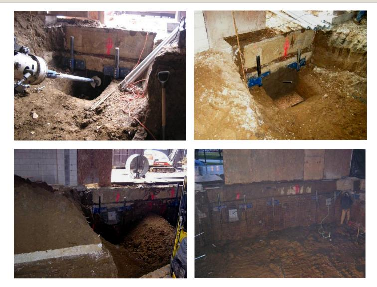
Another solution is to install tie-back anchors to brace the foundation at the top of the piles.
