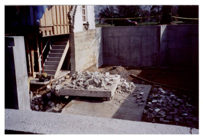
During installation of piers, the wall suddenly collapsed, tragically killing one of the workers.
