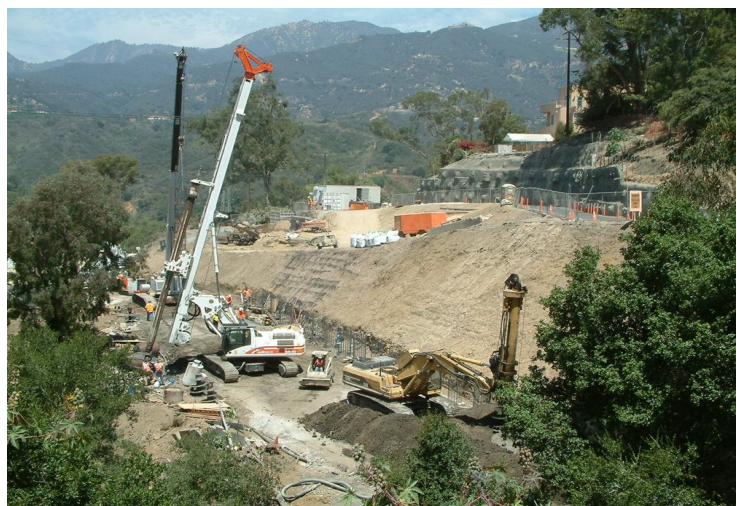
Figure 34 Construction of tied-back support walls designed by Cotton Shires.
