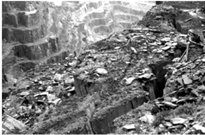
Figure 6 - Obsequent , or antislope scarps (uphill facing normal faults) that typically form by rotational extension behind a toppling face.
