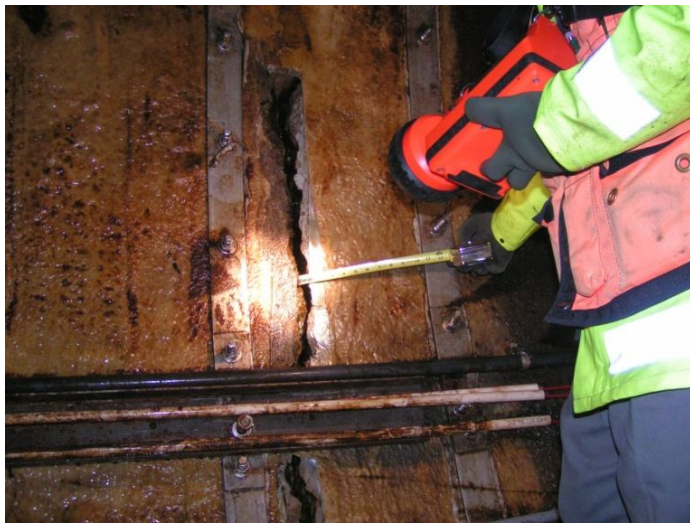
Fig. 29 One of the main cracks through the Belden Tunnel in 2006
