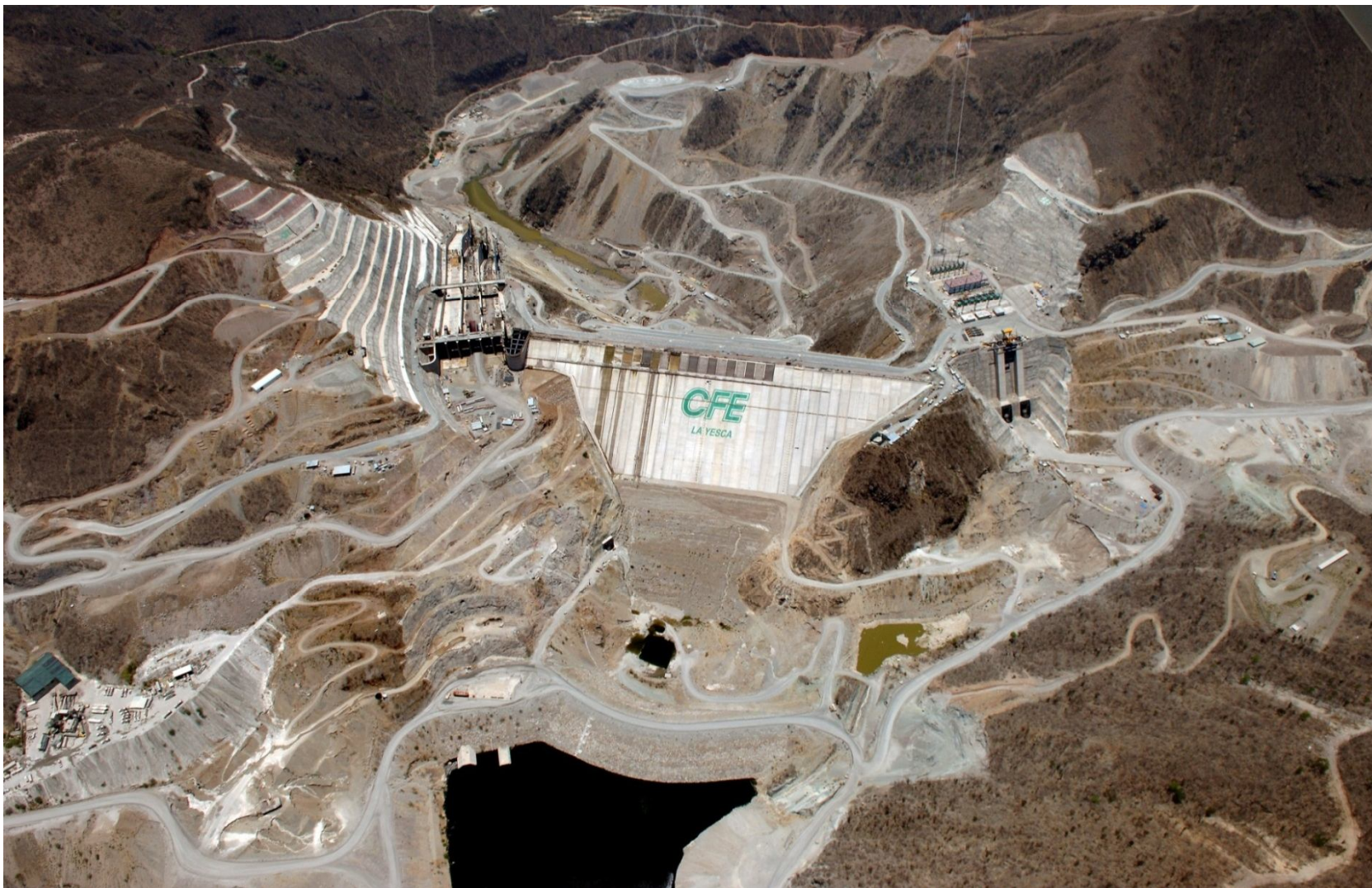
GENERAL VIEW OF THE DAM MAY-2012
