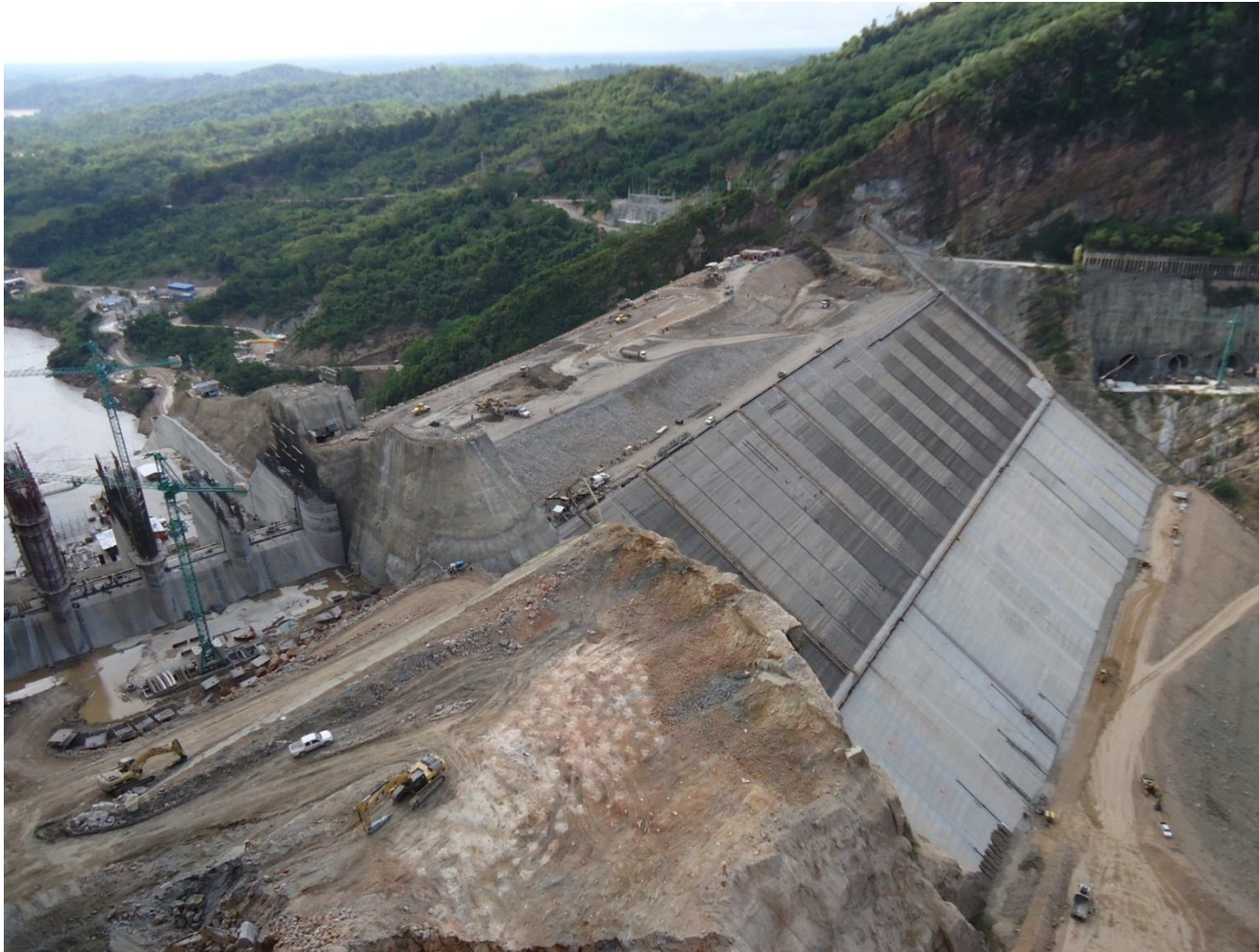
Panoramic view of the Dam. September 2013
