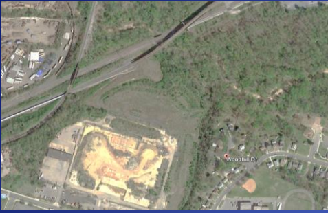
WMATA Slope Failure Investigation Cheverly, MD
