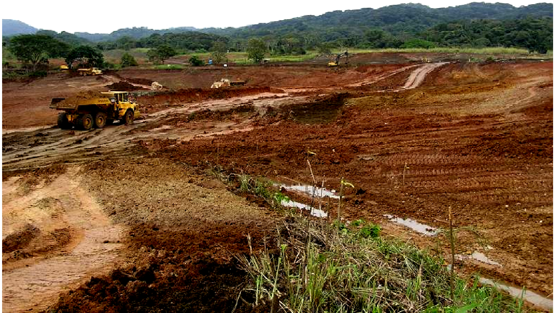
Excavation under way - late November 2005
