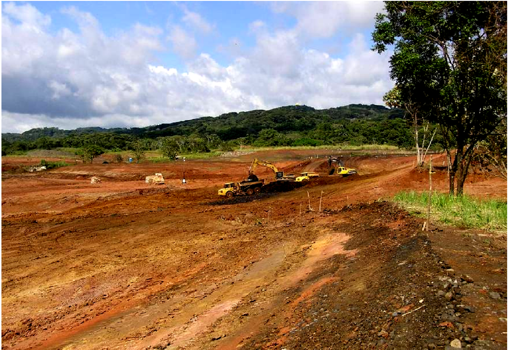
Excavation under way - mid-December 2005
