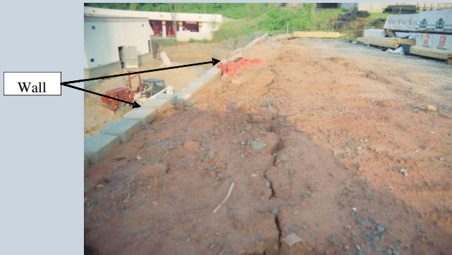
Tension Crack
