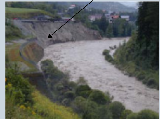
Adjacent River Flood
