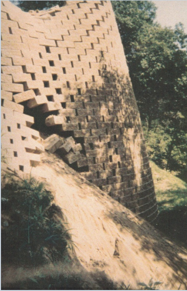
Saturated Backfill
