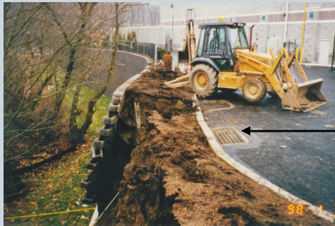
Surface water drainage inlet
