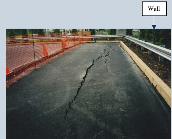
Tension Crack
