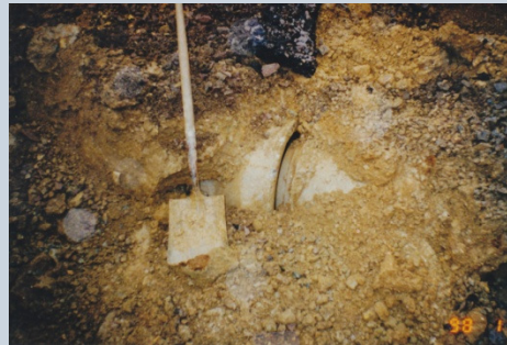
Surface water drainage inlet
