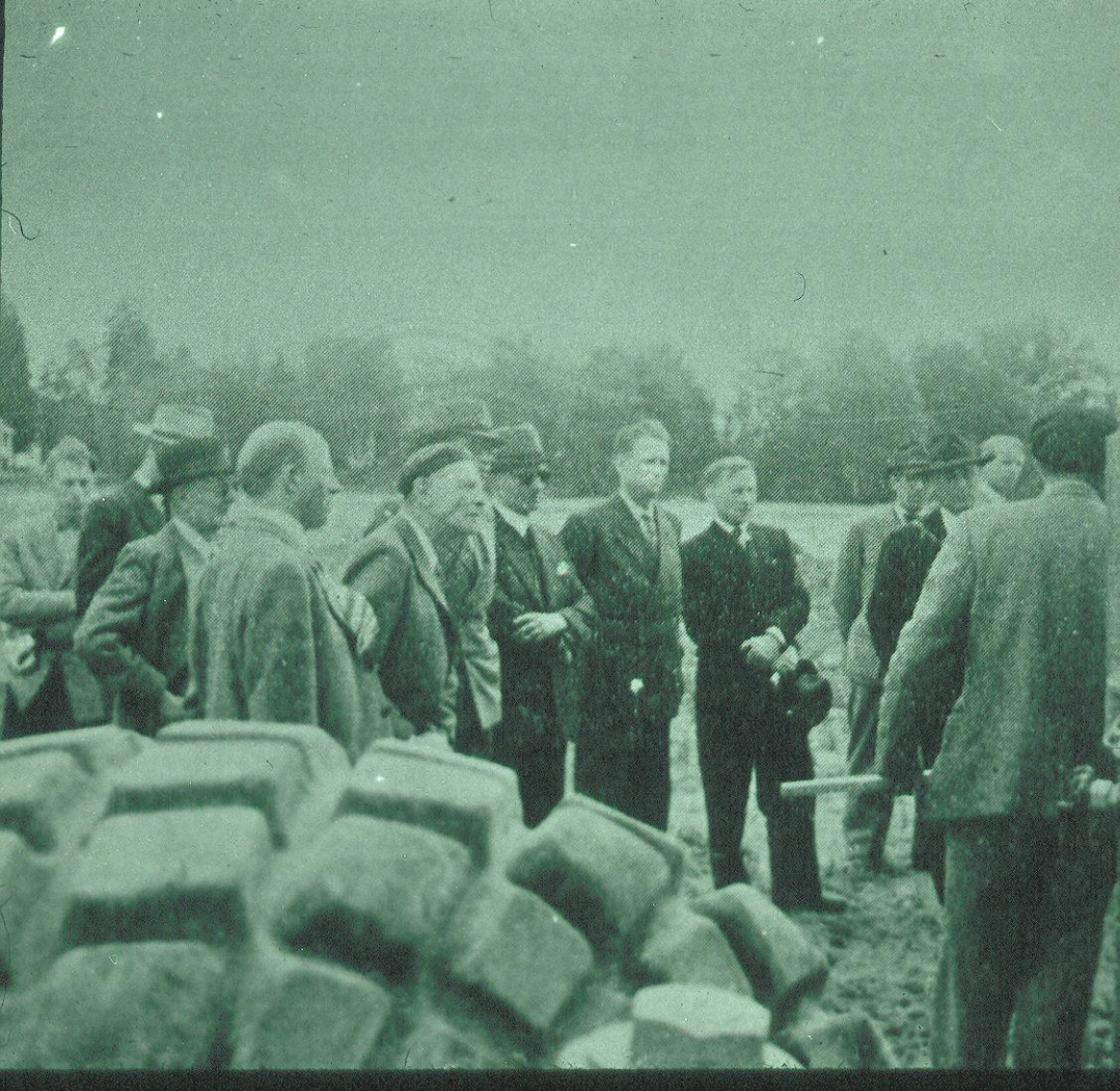
Kjellman paper drain installation, Halmsjön, Sweden, 1946 or 47?
