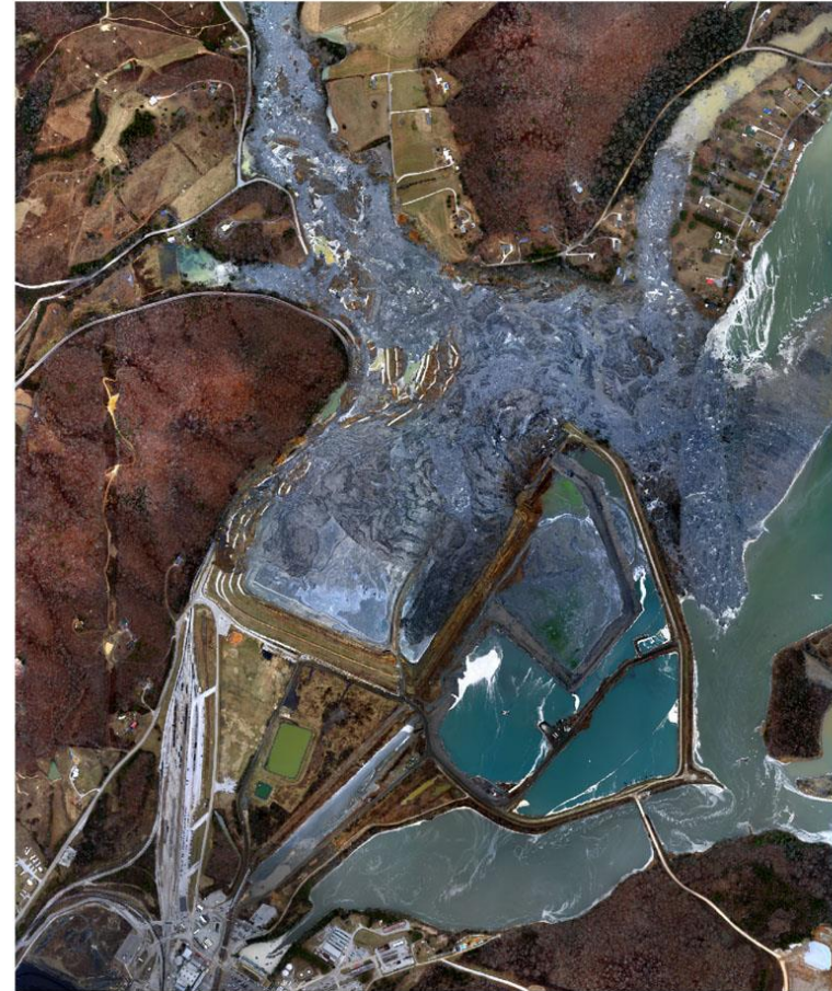
Aerial Image Of Kingston Ash Slide 12/23/08
