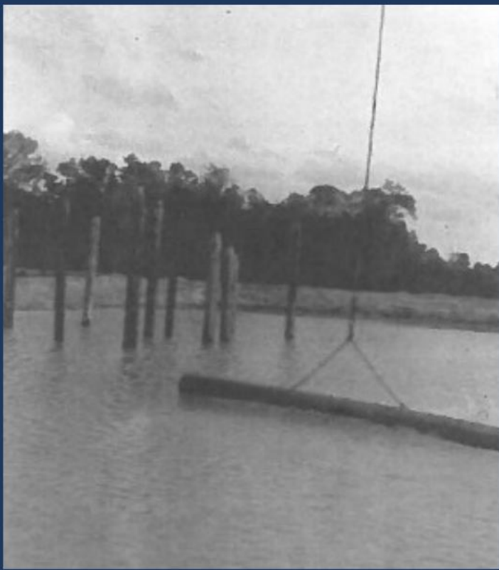
Connecting drainage pipe to sump platform
