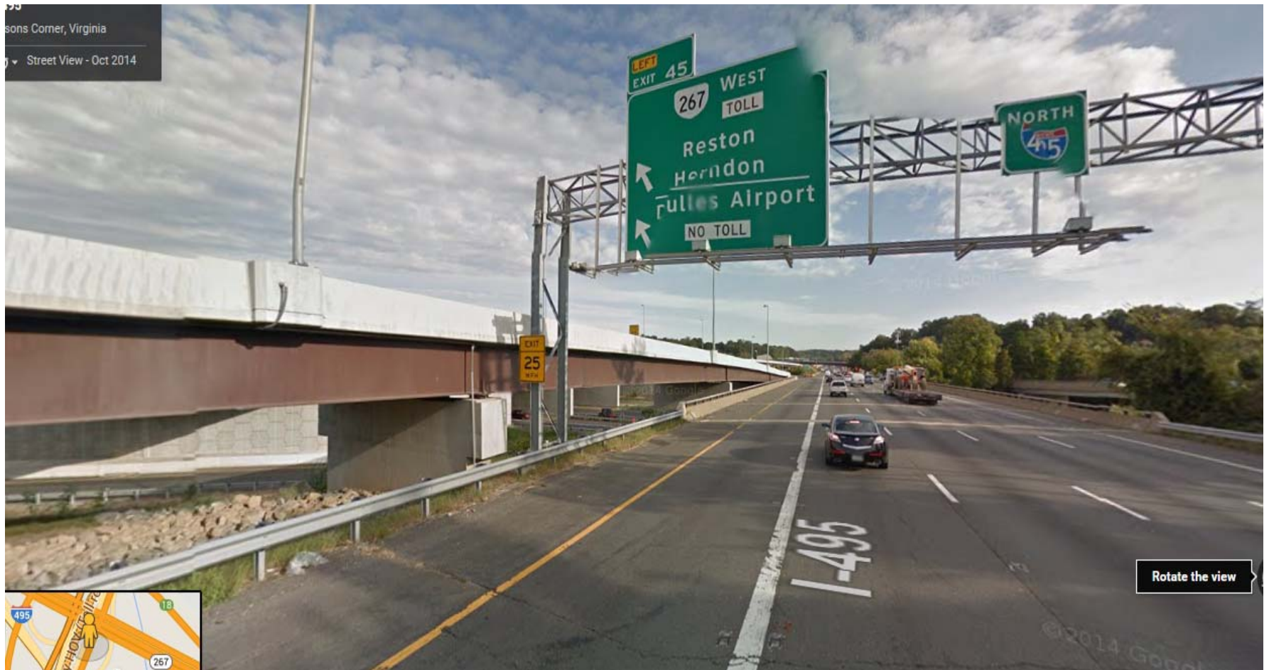
EXPRESS LANES VIADUCT OVER DULLES ACCESS ROAD
