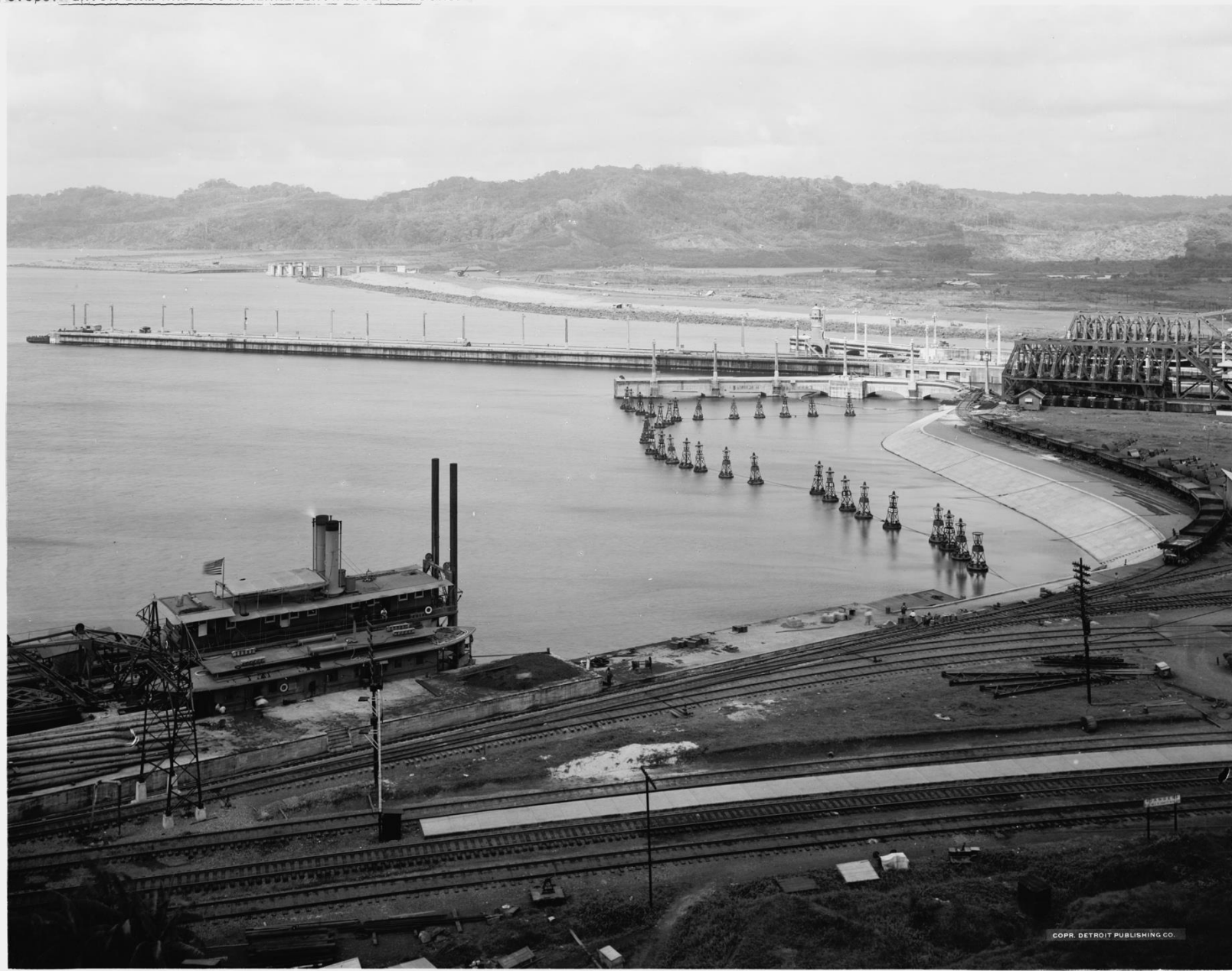
073307. GATUN DAM AND SOUTH (LAKE) ENTRANCE TO LOCKS.
