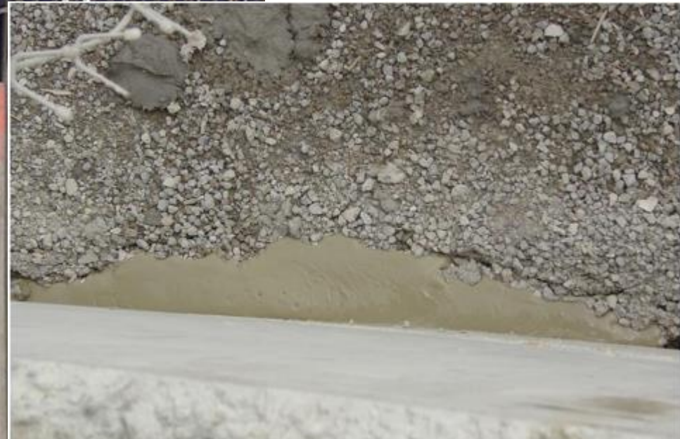
Results of injection (looking down from top of caisson)
