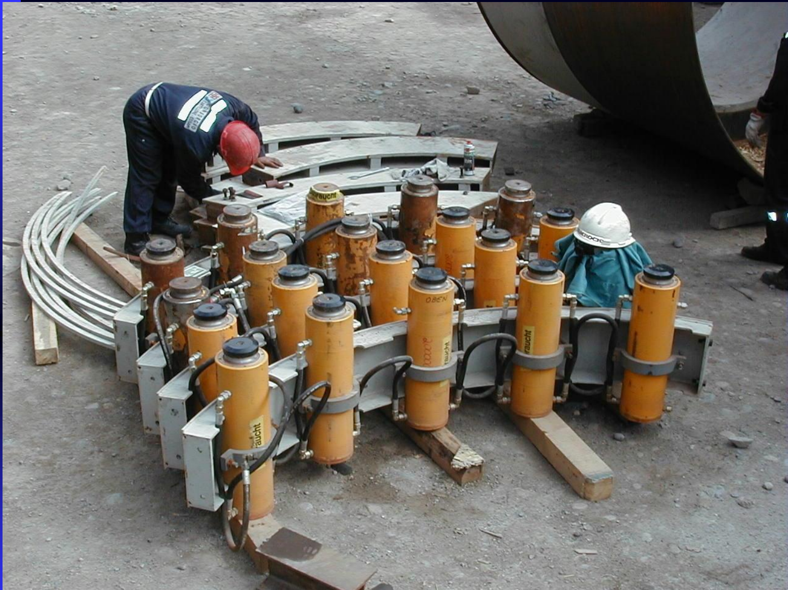
ASSEMBLY OF THE INTERMEDIATE JACKING STATION
