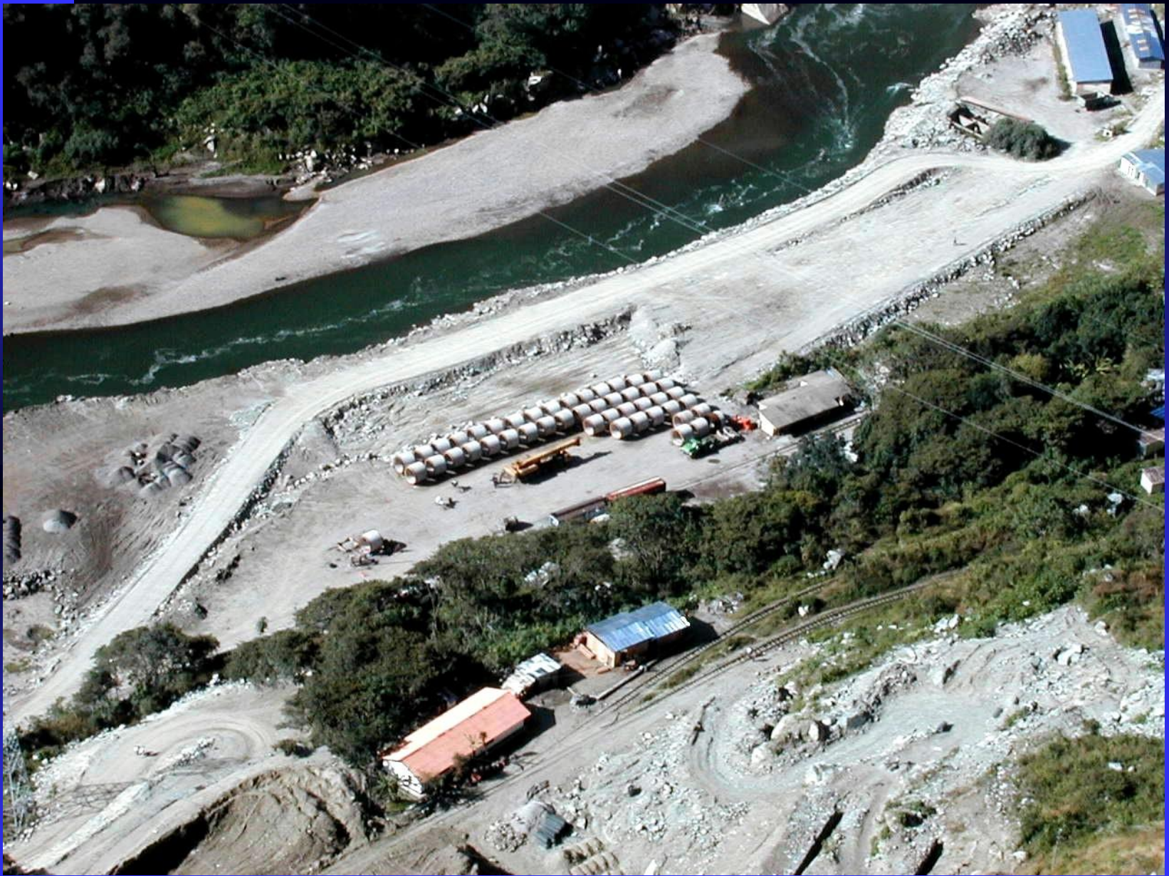
STOCK OF CONCRETE PIPES
