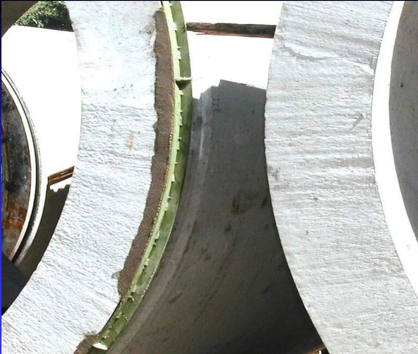
REPAIR WITH EPOXY MORTAR
