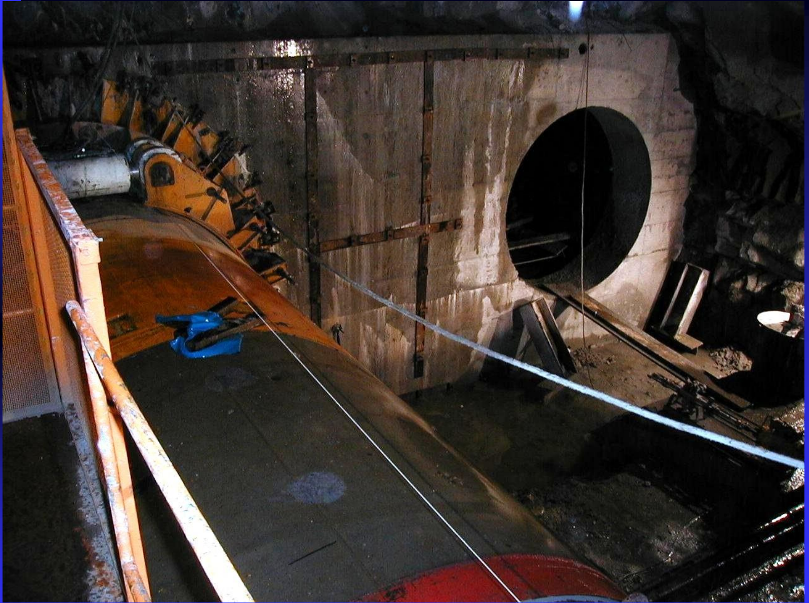
CAVERN OF RIGHT BANK
