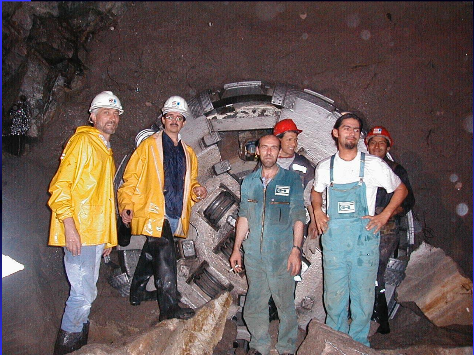
HOLE-THROUGH OF THE TUNNEL # 2
