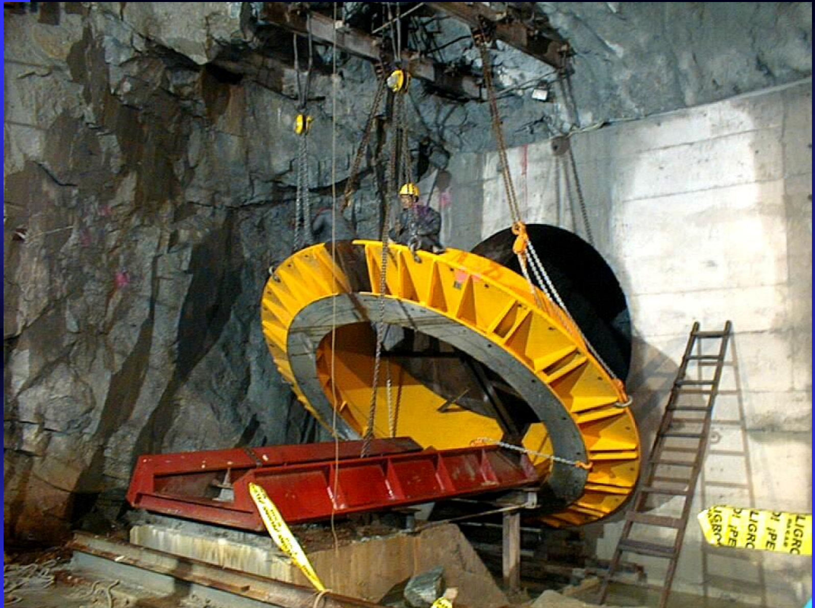
MOUNTING OF THE SEAL OF LAUNCH - TUNNEL NO.1
